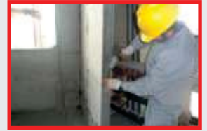
Anchoring upper panel to the lower
