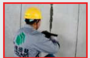
Filling up the mortar in clearance
